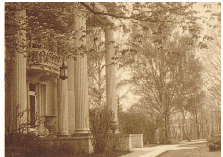
Ionic pillars on Hill-Bar (looking west).
