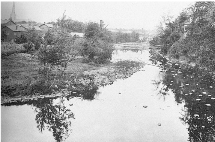
Prentice Swing Bridge 1896.
