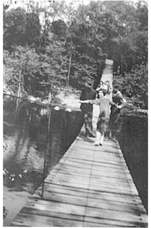
LaBounty Bridge north of Machpelah Cemetery.
