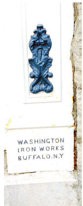
Details of iron work on Ross Block.
