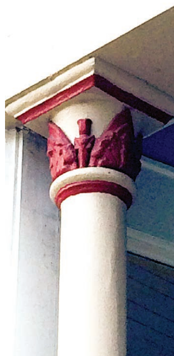
Top of iron column.
